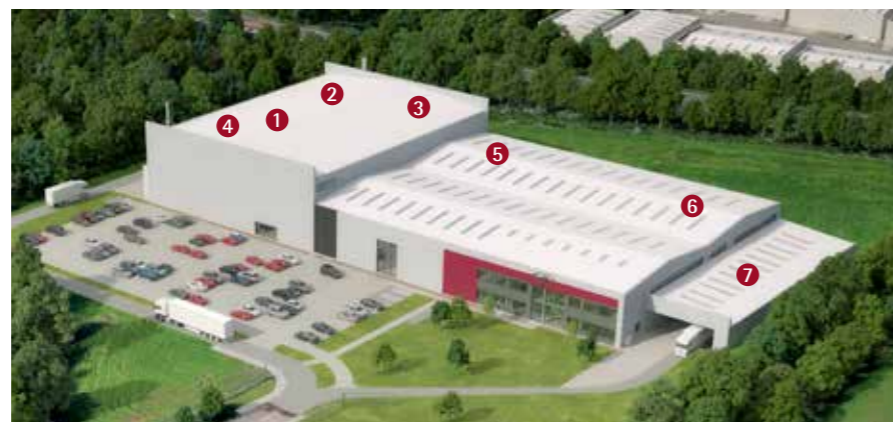
Overview of the production area of the future paint shop
