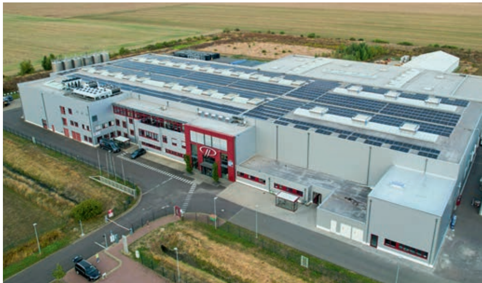
The photovoltaic system at POLYTEC's location in Wolmirstedt, Germany, delivers 614 kWp of power.
