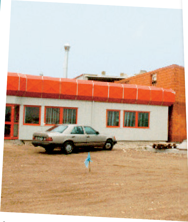
POLYTEC ELASTOFORM BUILDING UNDER CONSTRUCTION 1988
