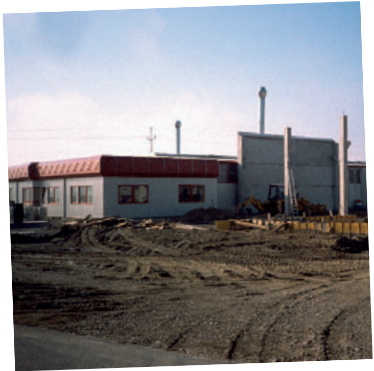
POLYTEC MARCHTRENK BUILDING UNDER CONSTRUCTION 1990
